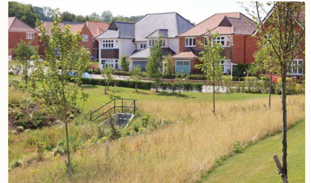
Generously planted Sustainable Drainage Systems within Marleberg Grange, Marlborough
