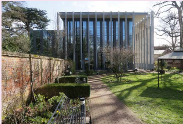
Bourne Hill Council Offices, Salisbury
