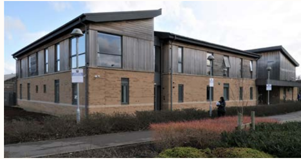
Trowbridge Health Centre
