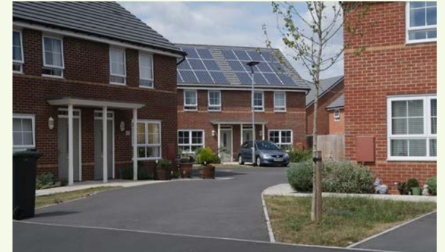
Owner-installed solar panels on south facing roof of new housing, Sandridge Place, Melksham
