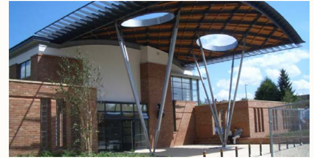
Wiltshire Police Station, Trowbridge
