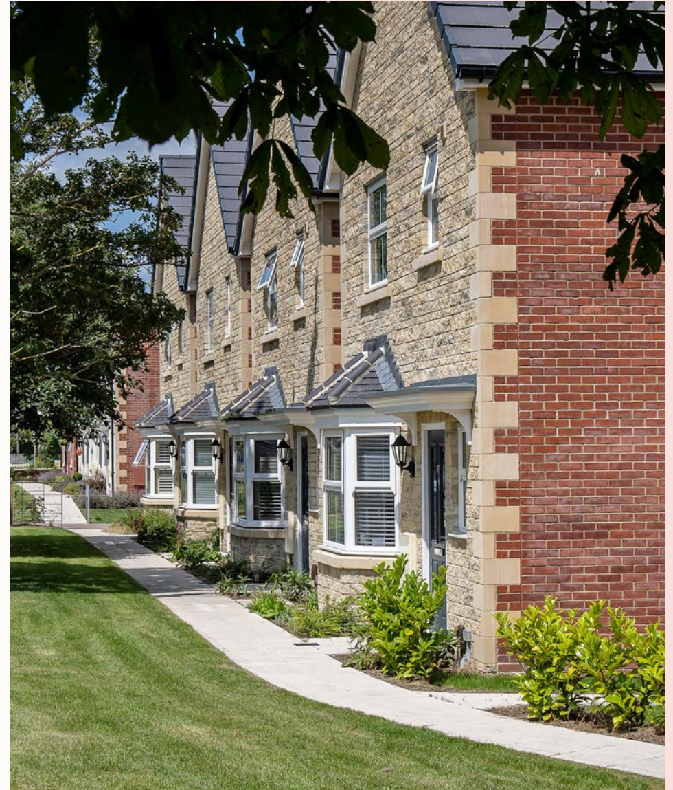
Newland Place, Trowbridge
